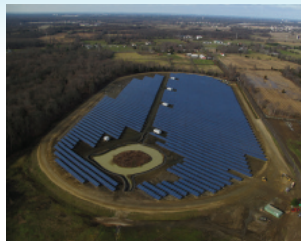
Medford Solar Inverter installation, an IBEW Local 351 project completed in December 2011.
