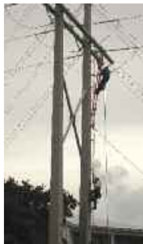
Orlando, FL, Local 222 members work under balmy skies.
