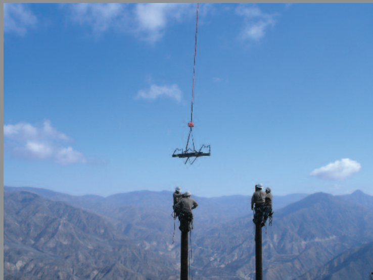
Tyrone Daum, Diamond Bar, Calif., Local 47 Daum documented four fellow members of the local waiting atop poles for a helicopter crossarm delivery after fires roared through the Los Angeles National Forest last year.
